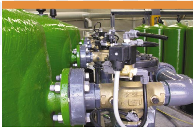
The TIRM plants are equipped with high quality valves for flow and backwash control.
