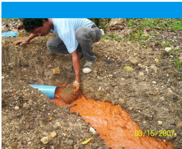
PolyVac Scourer Pipe End Retrieval
