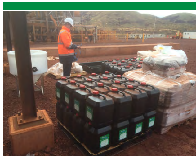
SCP removing bio-fouling from heat exchangers
